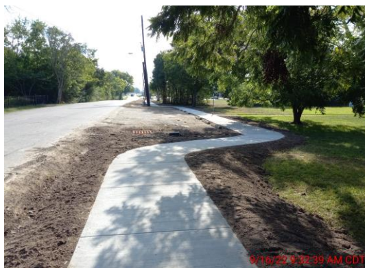
Figure 1: Newly constructed sidewalk September 16, 2022
