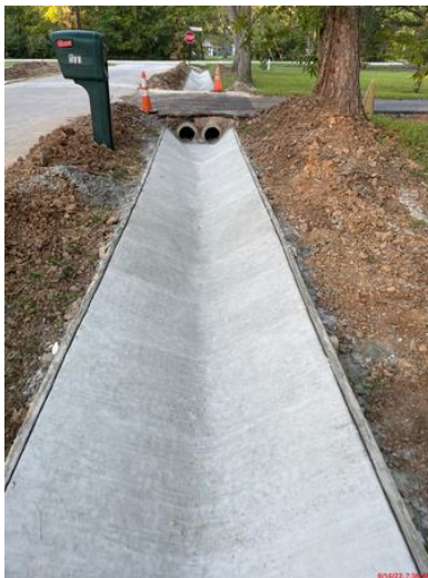
Figure 1: Newly constructed concrete lined ditch September 14, 2022
