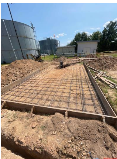
Figure 1: Generator pad formwork September 13, 2022
