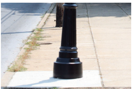
Acceptable Footer Detail
