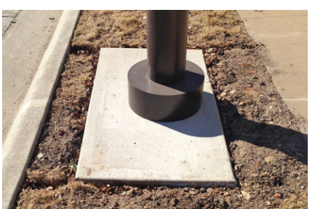
Acceptable Footer Detail
