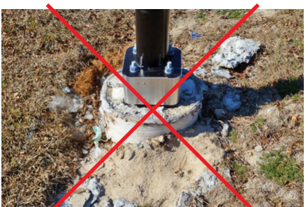
NOT Acceptable Footer Detail
