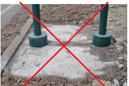
NOT Acceptable Footer Detail
