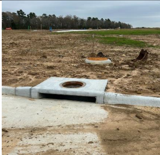
January 10, 2025 Storm Sewer Inlet Installation
