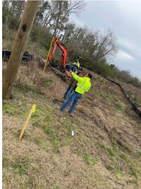
January 15, 2025 SWPPP Installation
