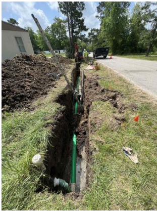
Figure 2: Sanitary Sewer Repair June 17, 2022
