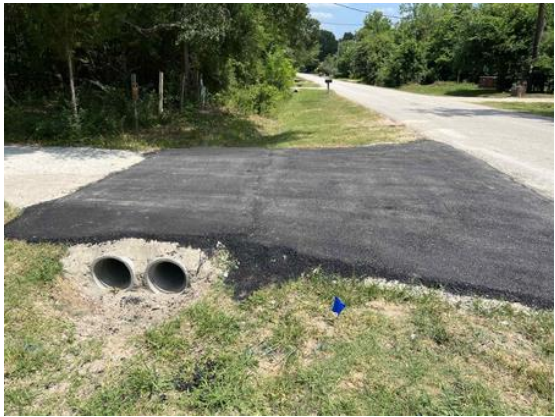
Figure 2: Culvert Replacement June 9, 2022
