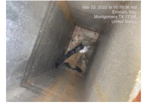
5-Remove SWPPP material from inside of inlet
