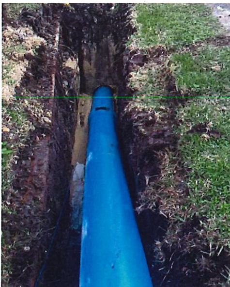
Trenchless construction on Pond St.
