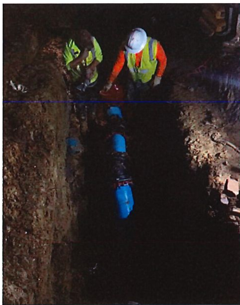
Overnight tie-in at SH-105 & Shepperd
