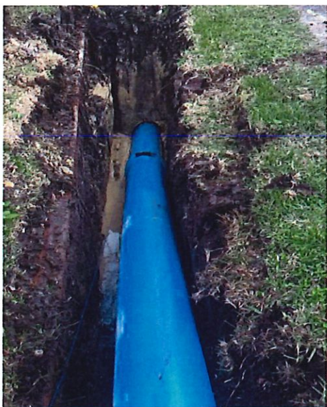
Trenchless construction on Pond St.
