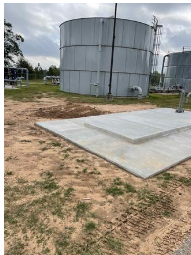
Figure 2: New Generator pad November 3, 2022
