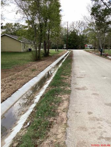
Figure 1: Newly Constructed Roadside Ditch along McGinnis November 15, 2022
