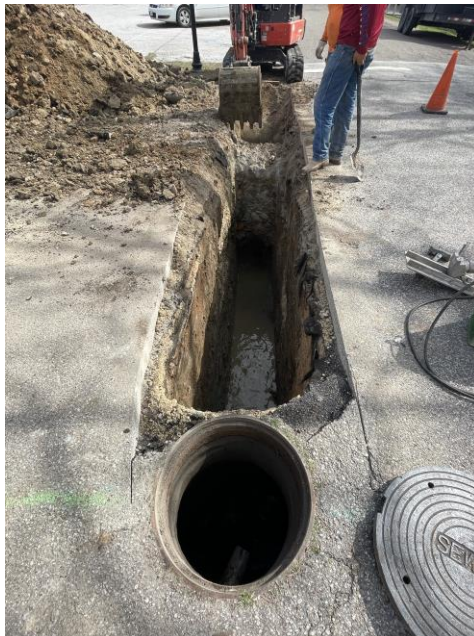
Figure 1: Point repair on McCown, February 6, 2023
