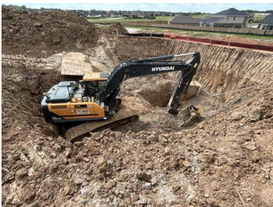
Excavation of the Lift Station wet well October 24th
