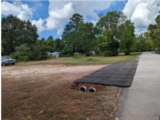
Figure 1: Culvert Replacement July 15, 2022
