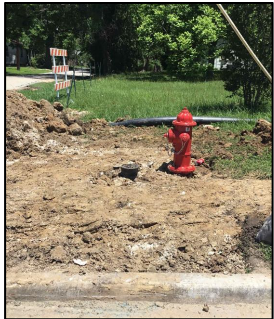
Flush Valve Install at SH-105 & Louisa St.
