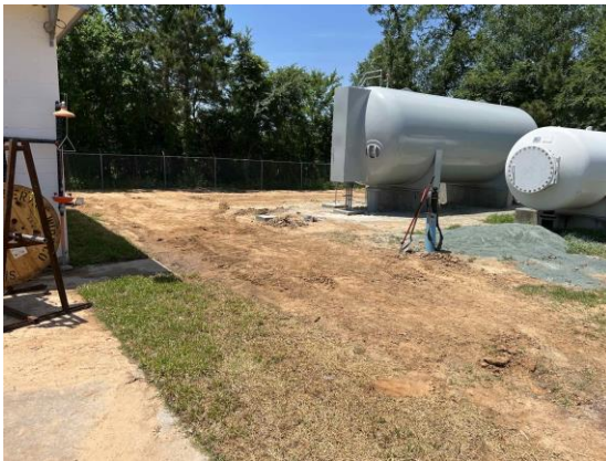
Figure 1: Hydropneumatic Tanks May 17, 2022
