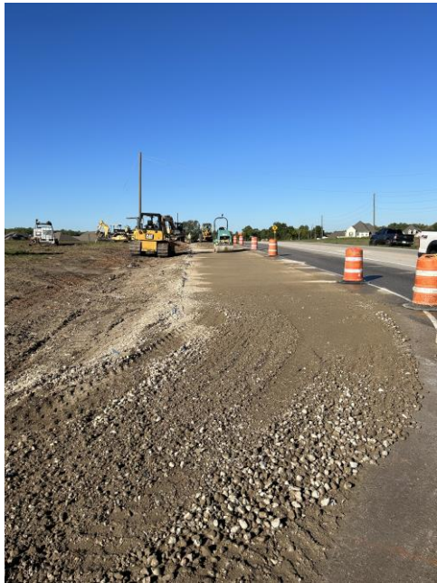
Subgrade Preparation (Westbound) October 18, 2023
