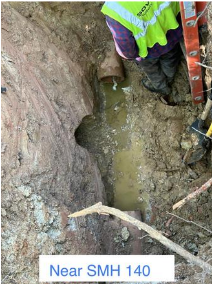
Point Repair to existing Sanitary Sewer Line October 13 th
