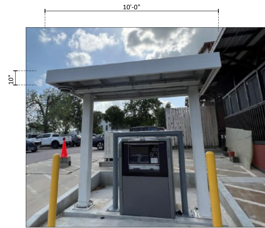
C3 EXISTING CONDITIONS TYPICAL FRONT / BACK
