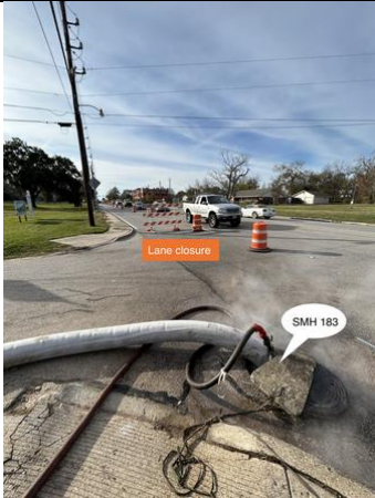
CIPP Lining at SH 105 and Louisa Street December 12 th
