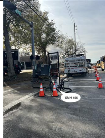
CIPP Lining along SH-105 on December 12 th
