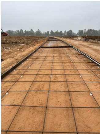
Formwork for proposed roadway January 18 th
