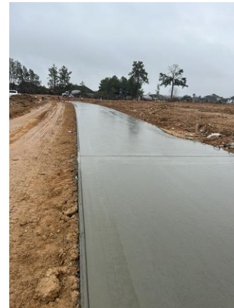
Formwork for proposed roadway January 18 th
