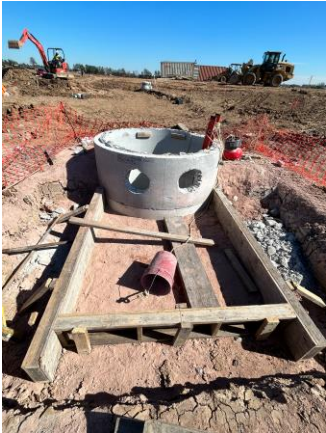
Well Head of the Lift Station January 17 th
