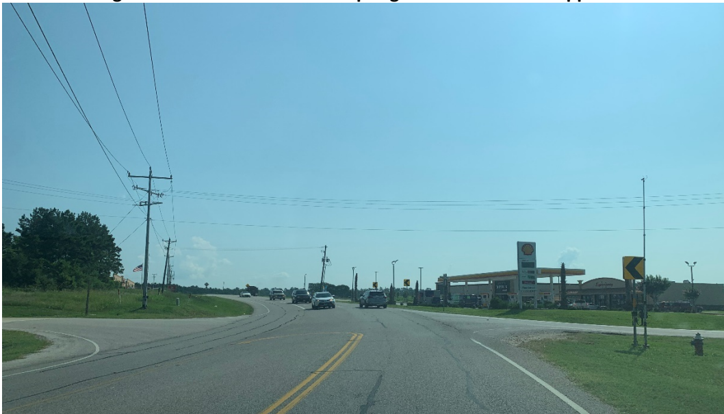
Figure 4 – FM 1097 at Buffalo Springs Drive Eastbound Approach
