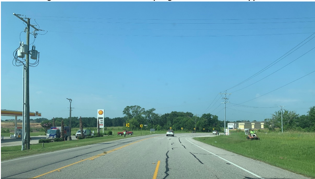
Figure 5 – FM 1097 at Buffalo Springs Drive Westbound Approach
