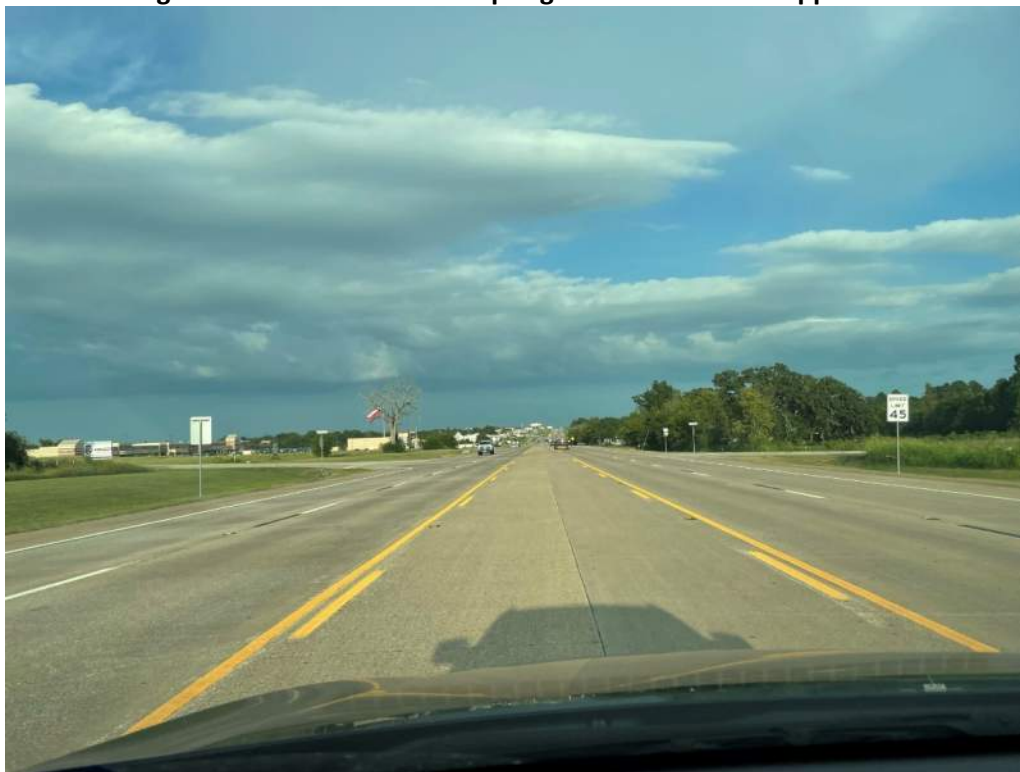
Figure 4 – SH 105 at Buffalo Springs Drive Eastbound Approach
