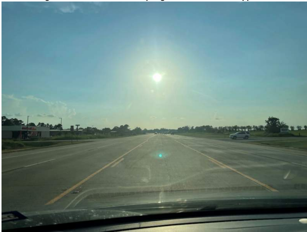
Figure 5 – SH 105 at Buffalo Springs Drive Westbound Approach
