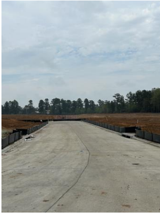
Roadway Paving March 15 th
