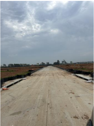
Roadway Paving March 15 th
