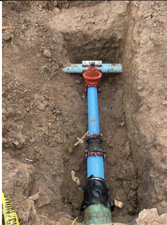
Figure 1: Installation of tapping sleeve and valve on April 18 th .
