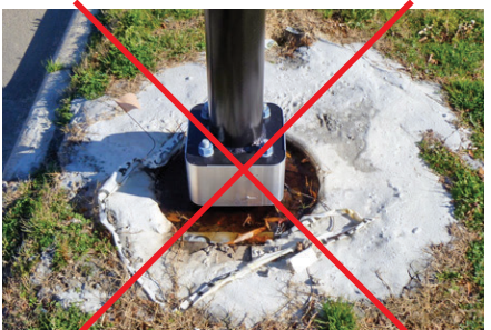
NOT Acceptable Footer Detail
