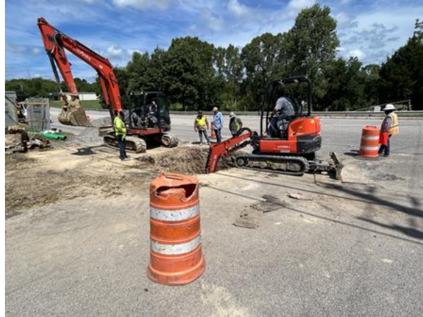
August 17, 2024 Sanitary Sewer Manhole Installation
