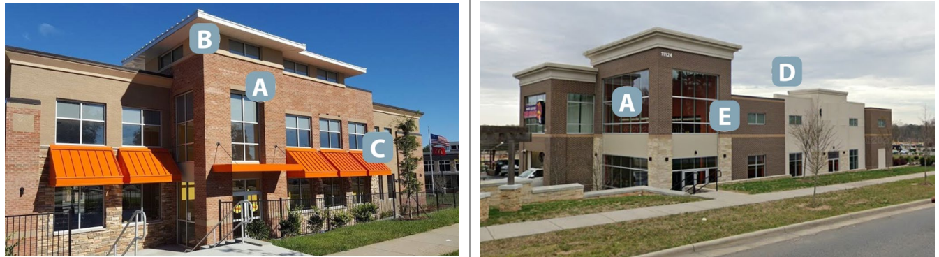
Figure Notes: A = Windows in Mid-section of Facade | B = Clerestory Windows | C = Shading Devices | D = Varied Rooflines and Parapet Heights | E = Change in Materials
