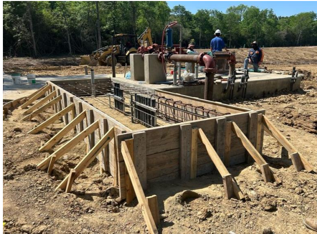
April 9, 2025 Briarley Lift Station Rebar Installation
