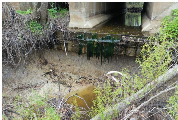
March 27, 2025 Plez Morgan Culvert Undermining
