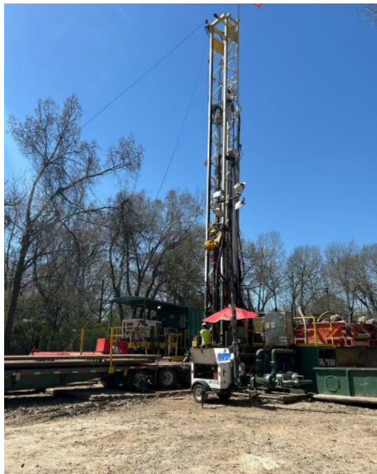
March 3, 2025 Well Drilling
