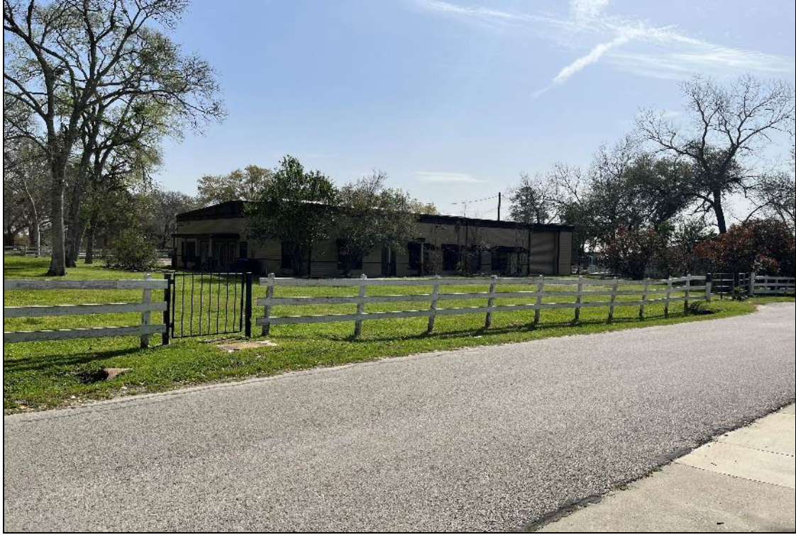
View of the subject property looking southeast across Maiden Lane
