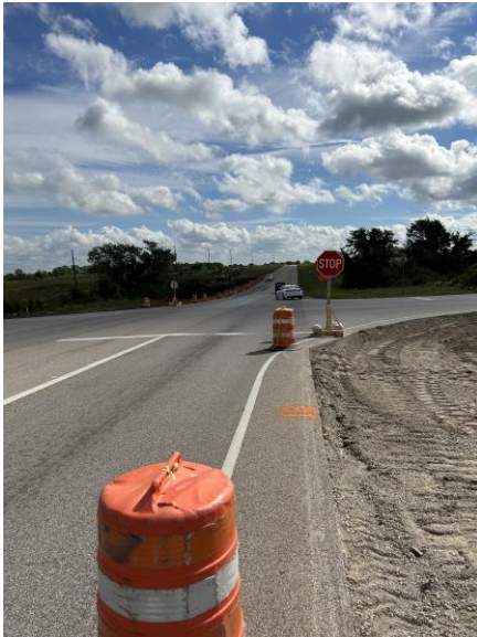
Subgrade Preparation (Eastbound) September 21, 2023
