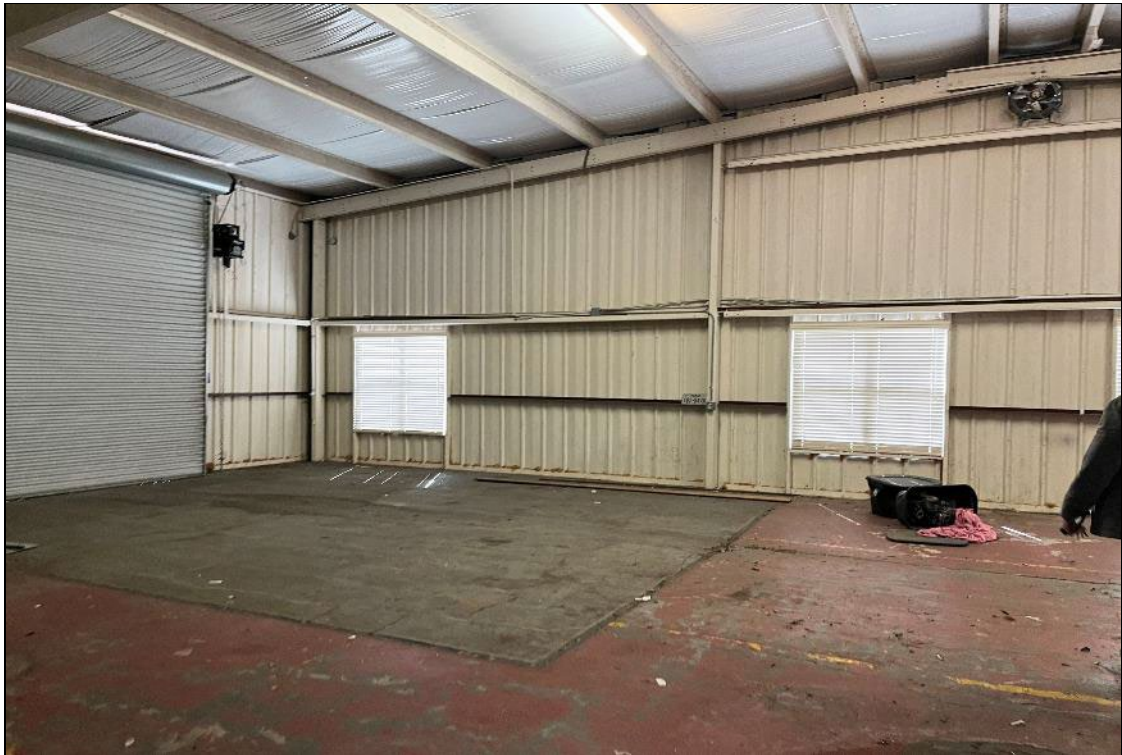
Interior view of the warehouse area
