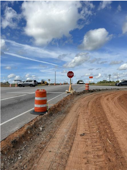
Subgrade Preparation (Northbound) September 21, 2023
