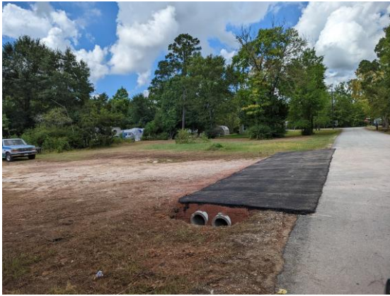
Figure 1: Culvert Replacement July 15, 2022
