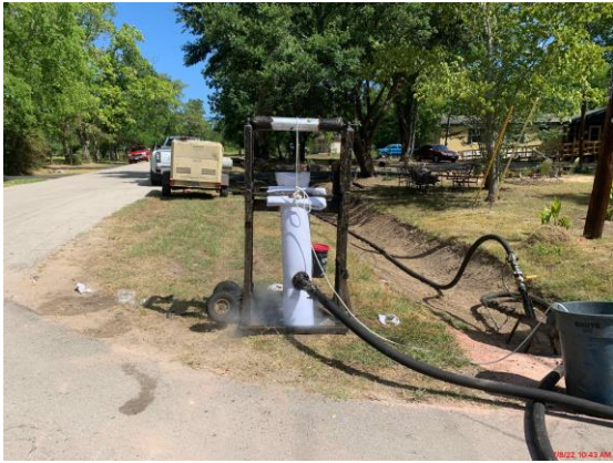
Figure 2: Sanitary Sewer CIPP Installation July 8, 2022
