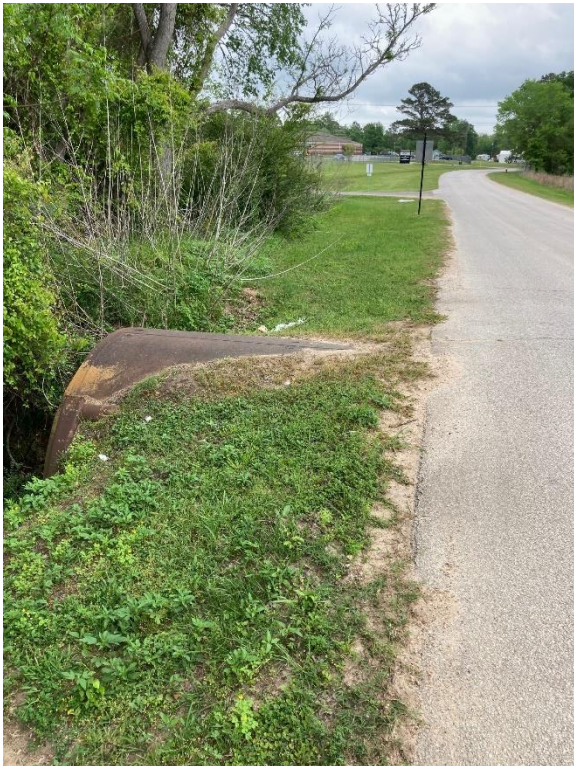
Existing 108" culvert at Anders Branch. Project calls for 10' extension.
