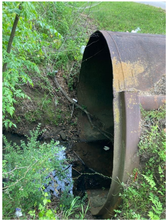
Existing 108" culvert at Anders Branch. Project calls for 10' extension.
