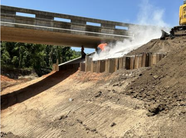
Lonestar Parkway Bridge construction July 19, 2023
