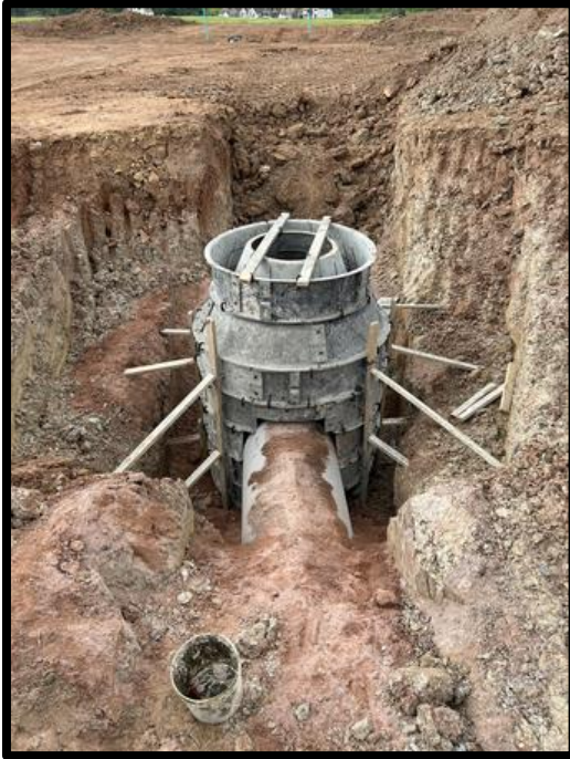
Storm Sewer Manhole installation July 6 th
