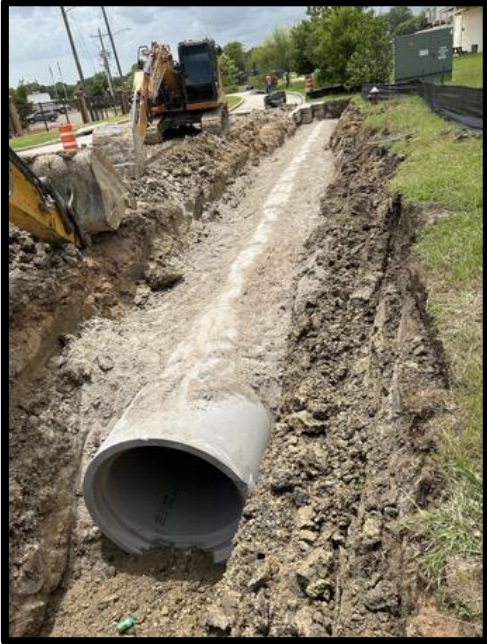
Storm Sewer Backfill on July 5, 2023
