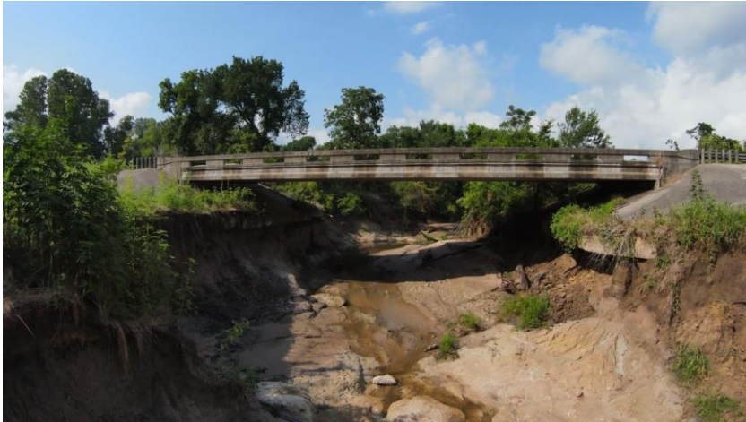
Lonestar Parkway Bridge prior to construction
