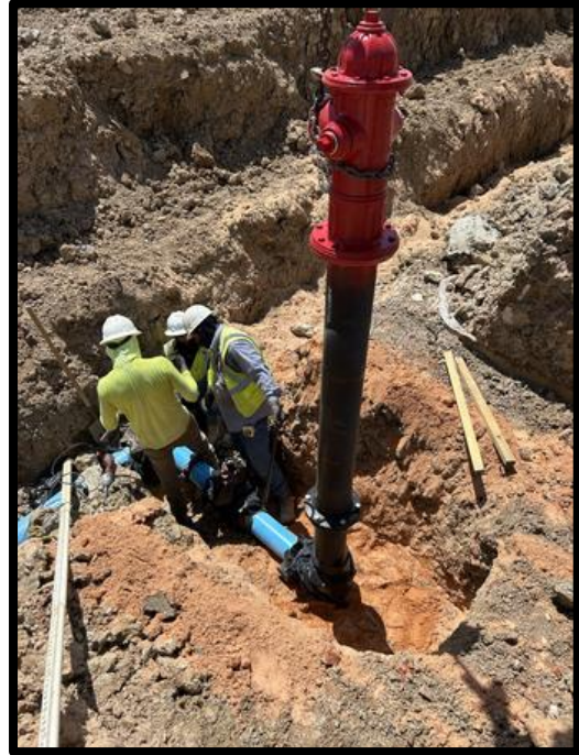
Waterline and Fire Hydrant installation July 13 th
