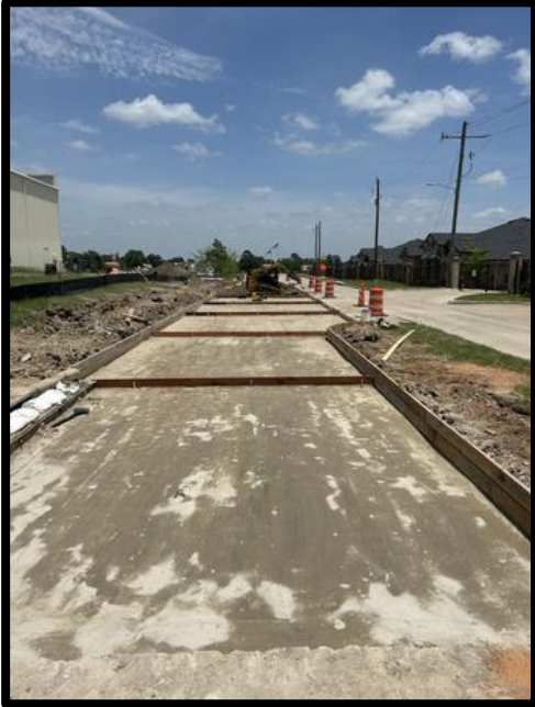
Pavement Formwork on July 14, 2023
