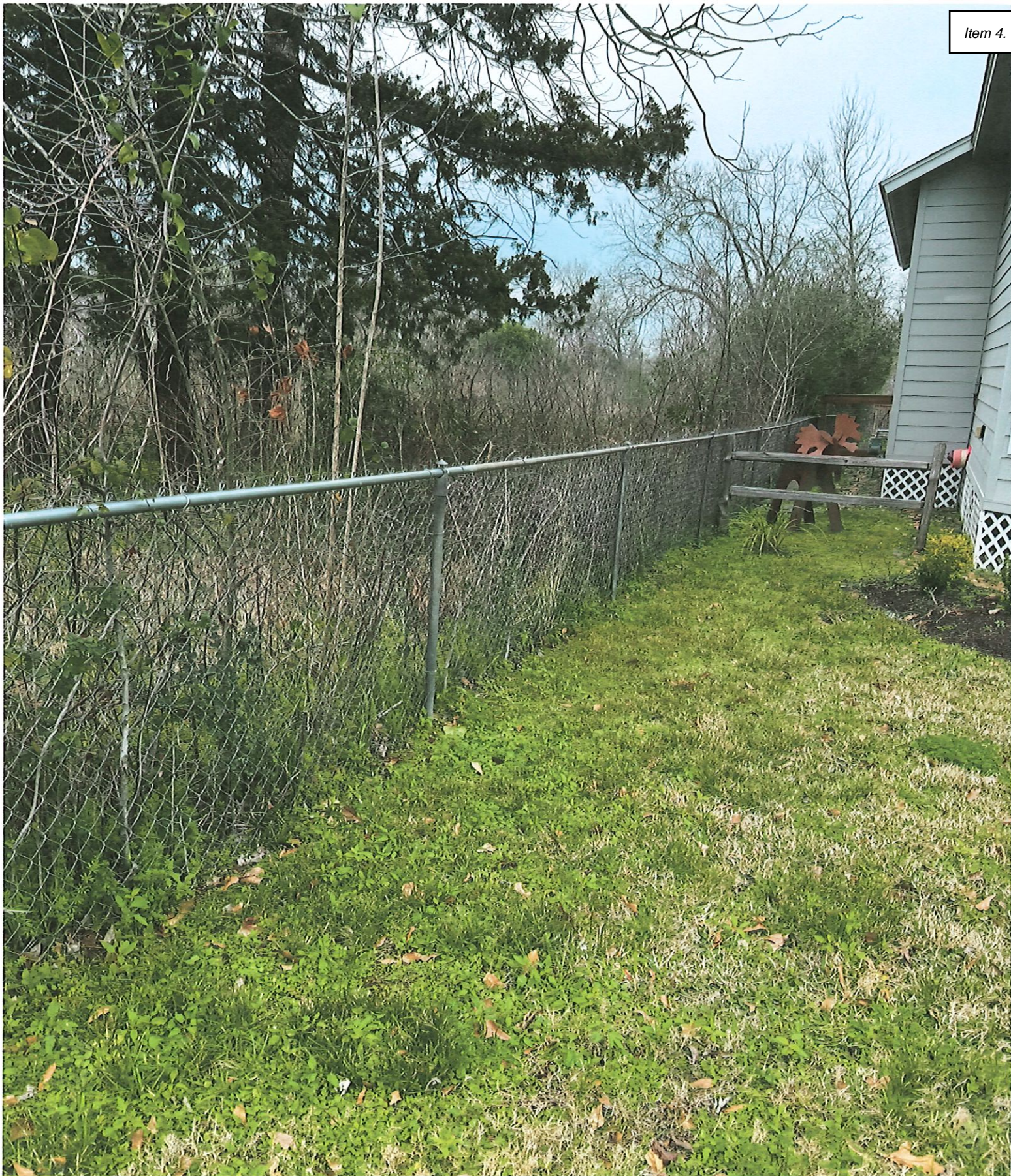
Current fence at front of property.
