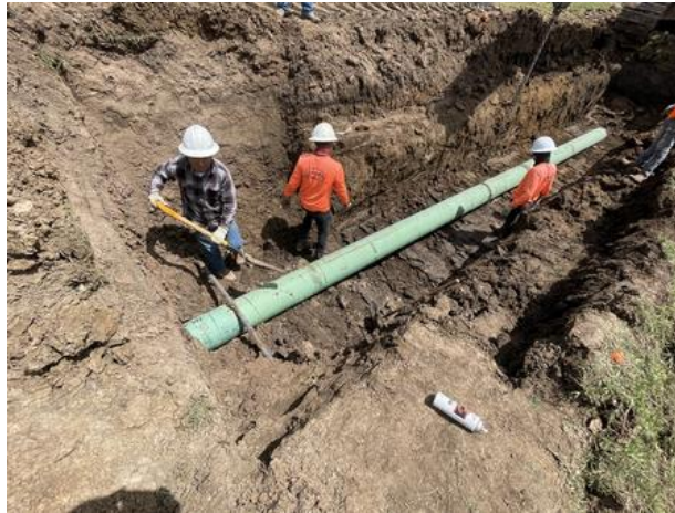
Figure 1: Installation of offsite waterline April 11 th
