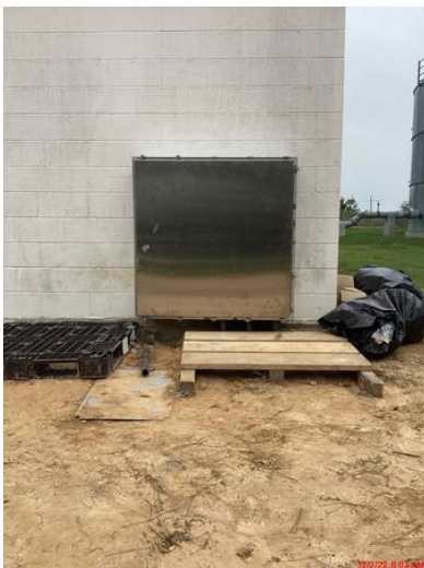
Figure 1: New electrical junction installed December 3, 2022
