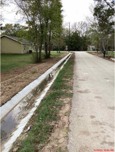
Figure 1: Newly Constructed Roadside Ditch along McGinnis November 15, 2022
