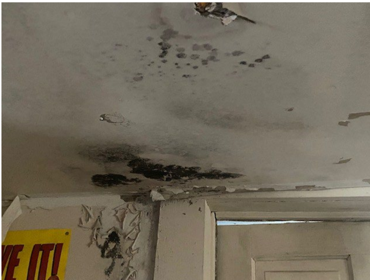
This is also located in the 2 nd addition.
