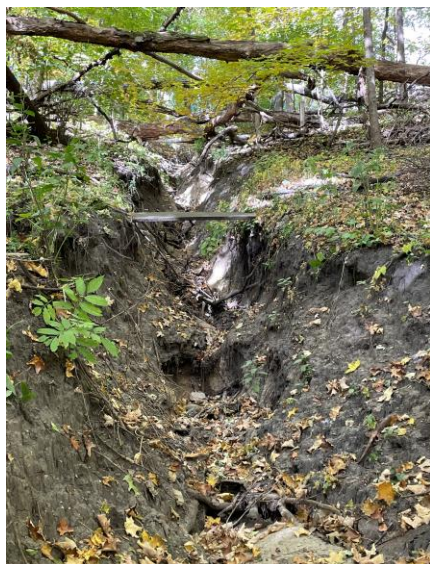
Figure 7. Erosion south of D'Chene Ln
