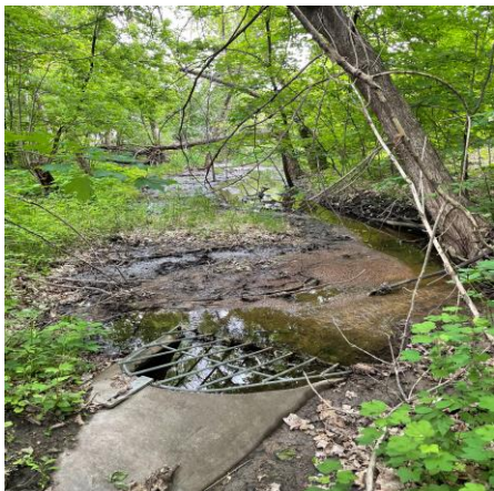
Figure 4. Storm sewer outlet at the southeast corner of CR 110 and CR 151
