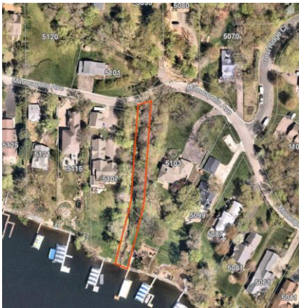
Figure 3. Fire Lane on Minneapolis Avenue
