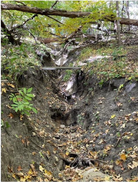
Figure 9. Erosion south of D’Chene Lane
