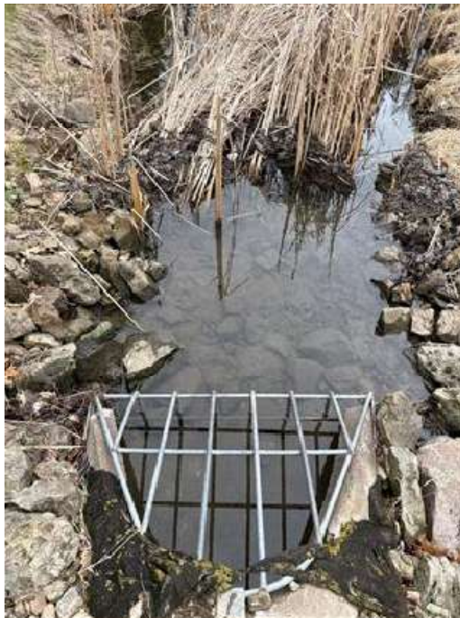
Figure 3: 18" RCP Inlet (N)
