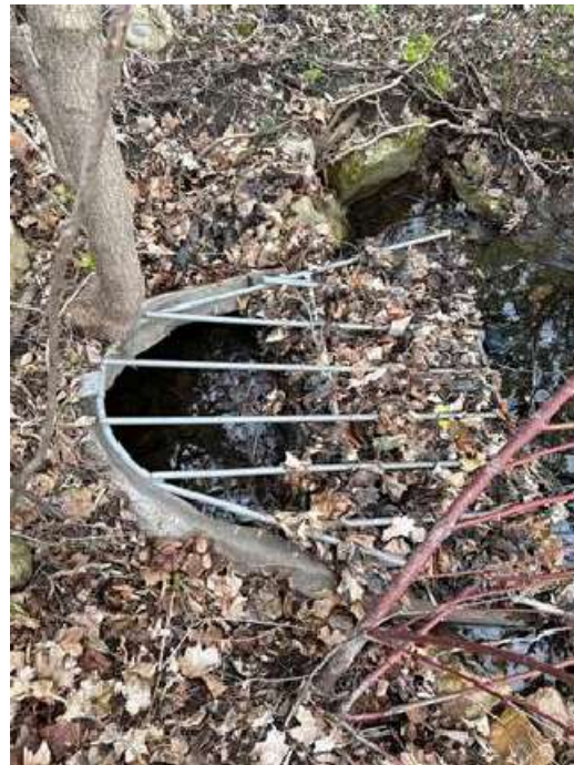
Figure 9: 24" RCP Inlet (S)
