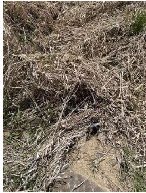
Figure 2: 12" RCP Outlet (NE)
