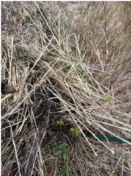
Figure 8: 15" RCP Inlet (NE)
