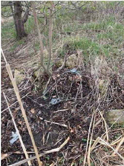
Figure 14: 15" RCP Inlet (S)
