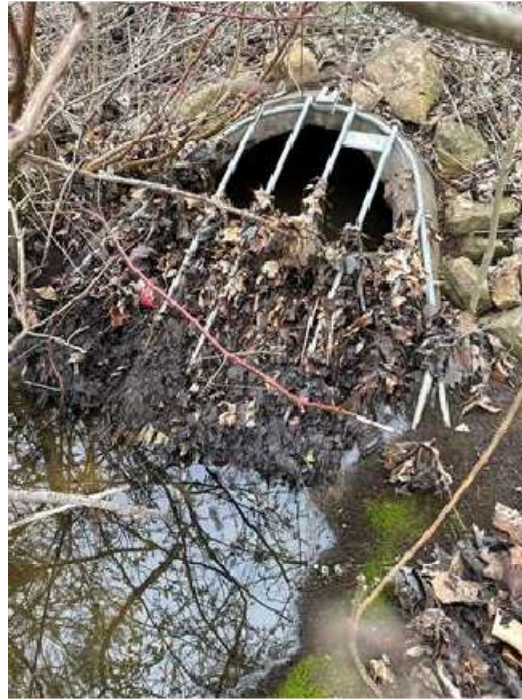
Figure 7: 24" RCP Inlet (N)
