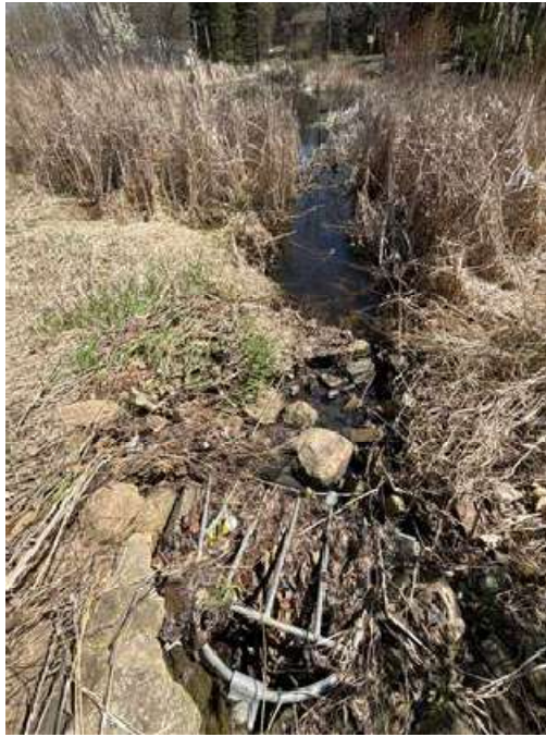
Figure 1: 18" RCP Inlet (SW)
