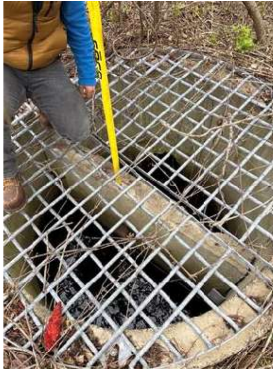
Figure 10: Outlet Control Structure (NW)
