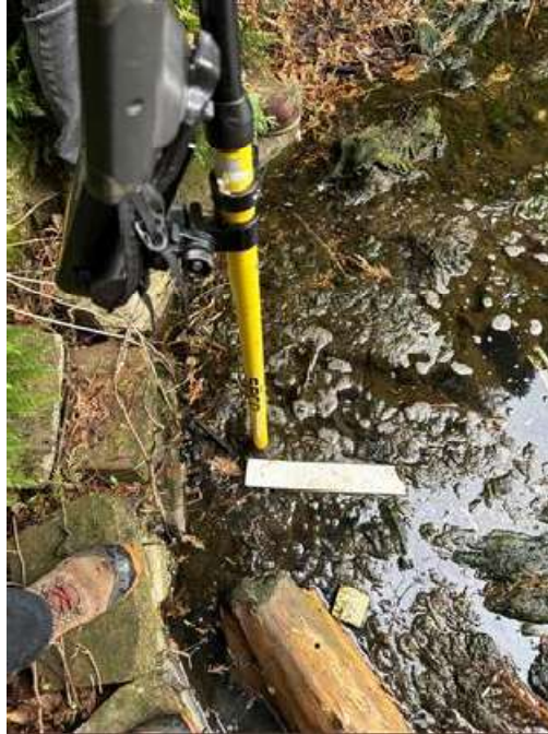
Figure 13: 12" RCP Outlet (S)
