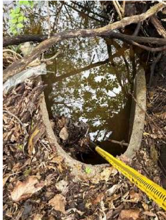
Figure 12: 15" RCP Inlet (SW)
