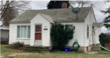
Lot #1 - Existing home is approx. a 1,000 sq. ft. footprint (picture above).
