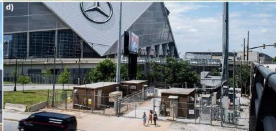
d) An edge data center by the Atlanta Mercedes-Benz Stadium in the city center - #3
