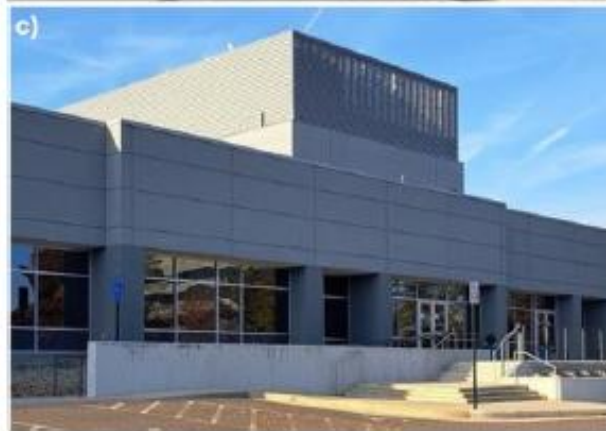
c) A CoreSite Colocation Data Center, Virginia - #4
