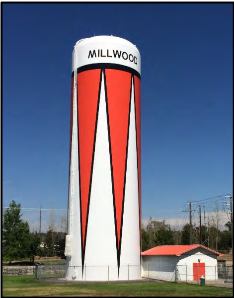
Figure 11-2: Millwood Water Tower
