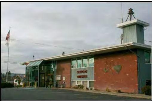
Figure 11-3: Millwood City Hall
