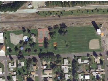
Figure 11-9: An aerial view of the Millwood Park
