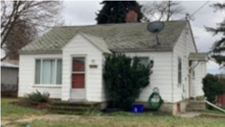
Lot #1 - Existing home is approx. a 1,000 sq. ft. footprint (picture above).
