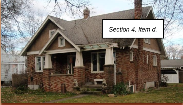
Stevens House, 3306 N Dale Rd
