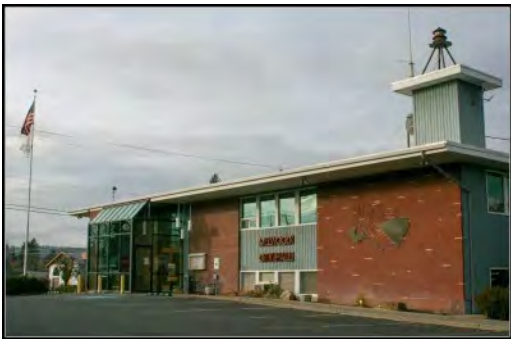
Figure 11-3: Millwood City Hall
