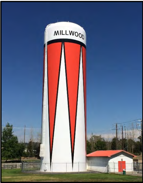
Figure 11- 12 : Millwood Water Tower
