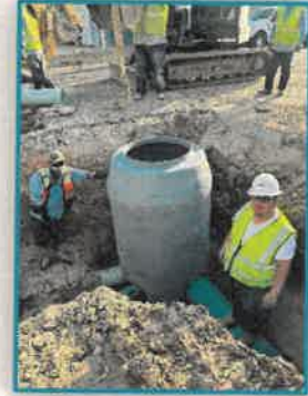
Dunlap / 1 st - Replaced Manhole
