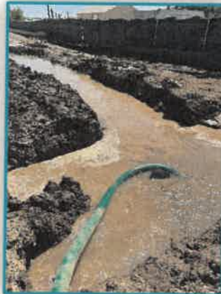
Conway / Military Repair of Water Break
