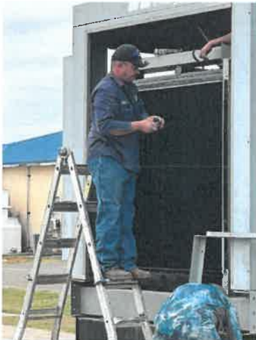
Emergency Generator Radiator Replaced
