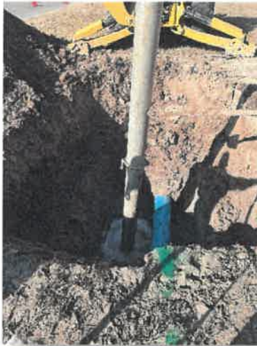
28 th /Conway Sewer Line Repair
