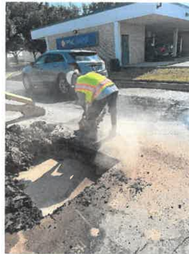
Conway/Bus 83 Water Line Repair
