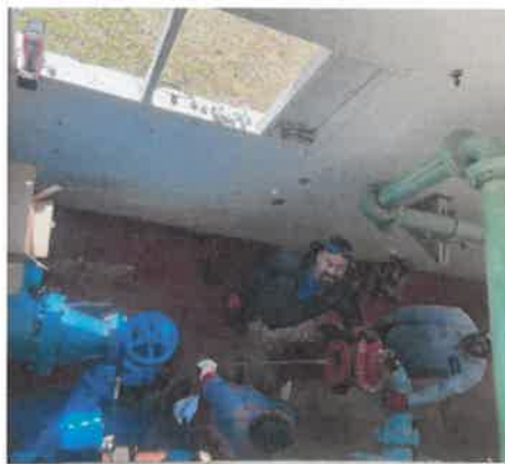
Backflow Preventer Check Valves Replaced
