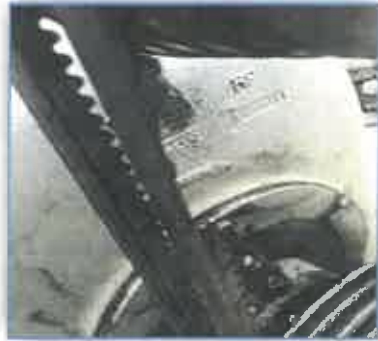
Lift Station Pumps Old Belt Replacement
