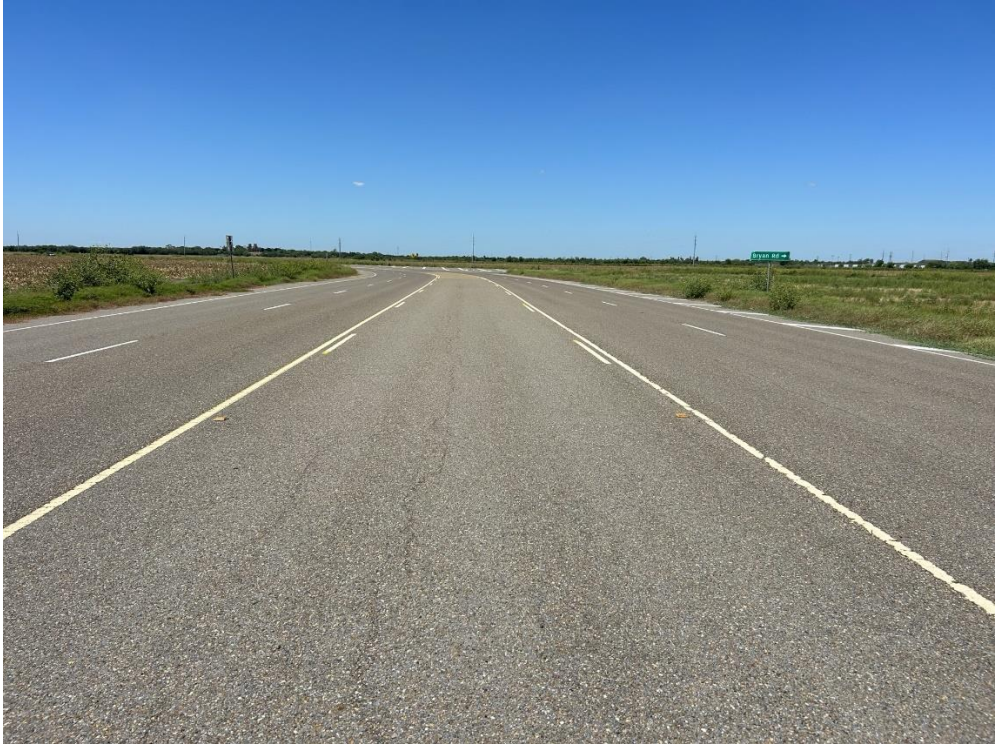
San Mateo Road looking West to Bryan Road
