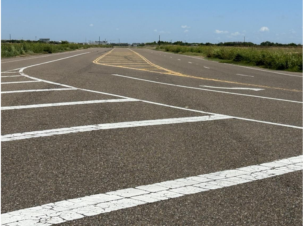
Intersection of San Mateo looking North on Bryan Road to Los Indios Road
