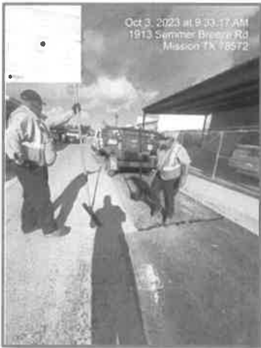
Summer Breeze Road Maintenance
