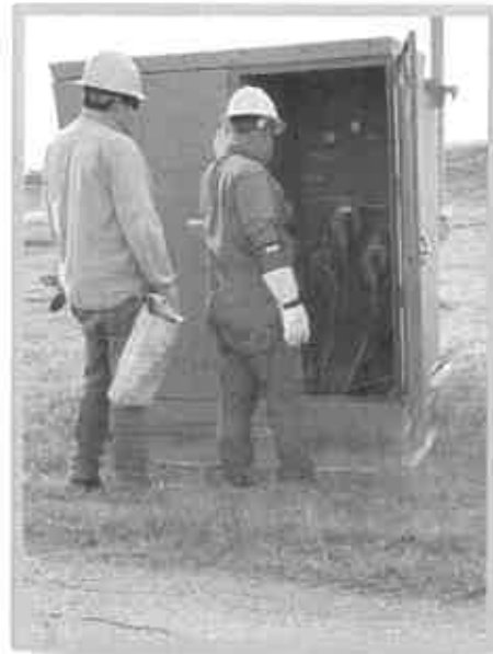
AEP Checking Electrical Surges
