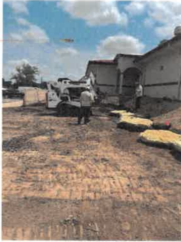
Placement of Retaining wall with boulders from Bannworth Park Pond / Irrigation Mainline Installation
