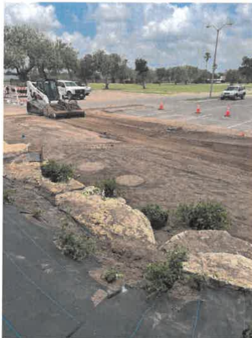
Soil Prep with Power Rake for the Preparation of New Lawn
