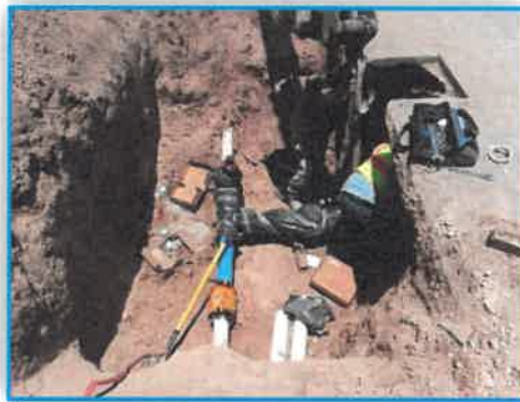
Amber Grove - 8 Inch Water Line Connection
