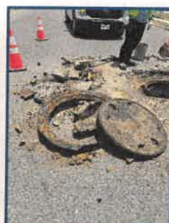
East 1 st Street Manhole Water Break Repair
