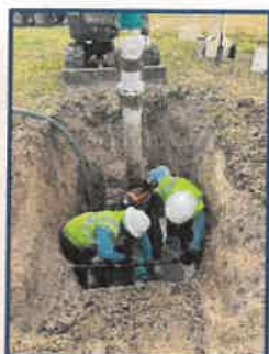
201 Melba Carter Hydrant T-Line Break Repair
