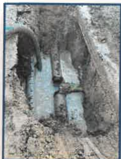
201 Melba Carter Hydrant T-Line Break Repair
