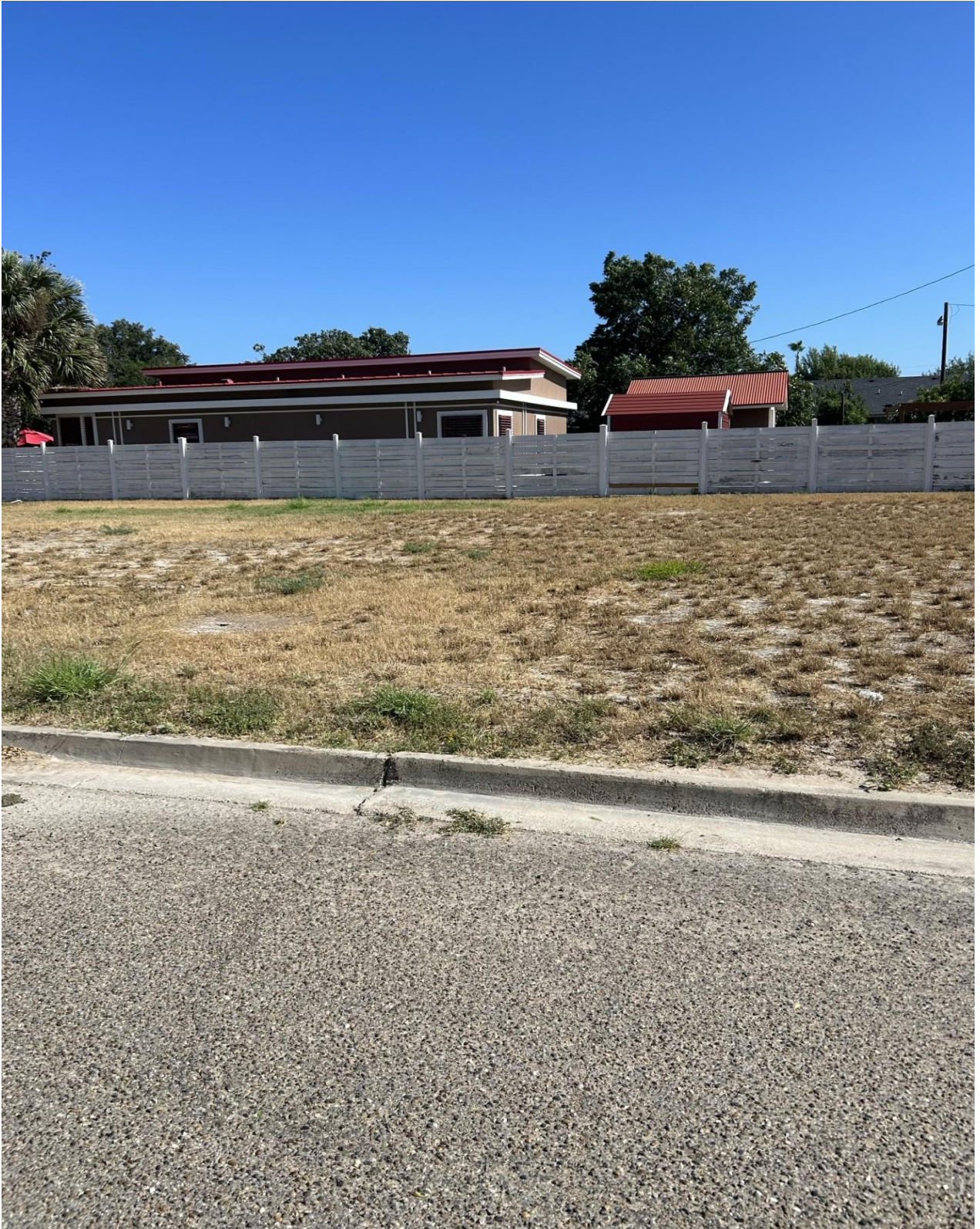
PHOTO OF THE SUBJECT PROPERTY FROM 4 TH STREET
