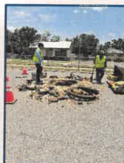
East 1 st Street Manhole Water Break Repair
