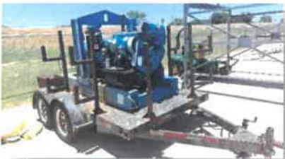
8-Inch Trash Pump Repair
