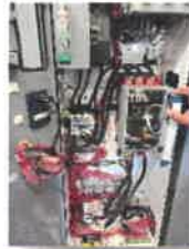
Lift Sta. Pump 6 Maint.
