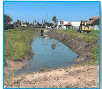
K-Mart Drain Ditch Long Reach Excavator Clean Out
