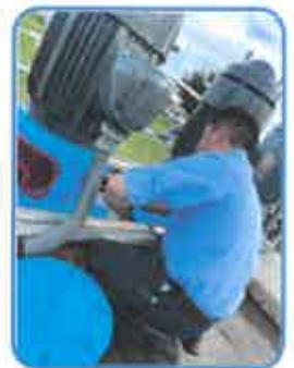
Train C Transfer Pumps Coating NWTP
