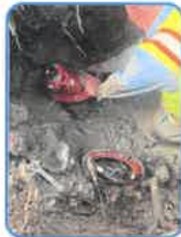
Replaced 2 Valves for Sludge Drain SWTP
